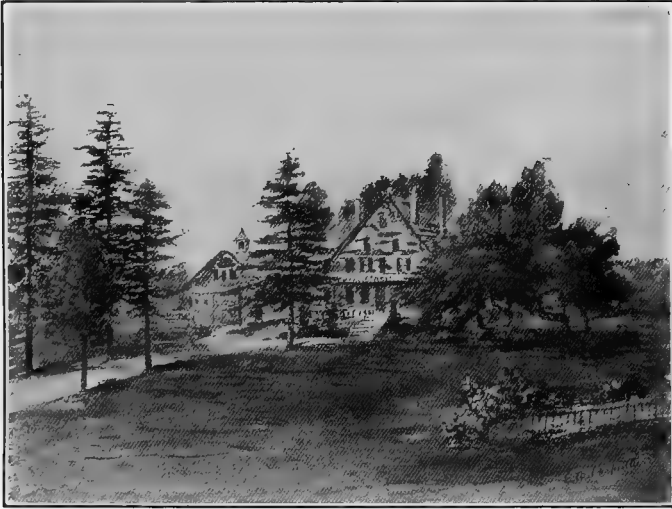
ESQUIRE FARWELL, OR JOHN O'CONNELL HOUSE, MAPLE STREET.
